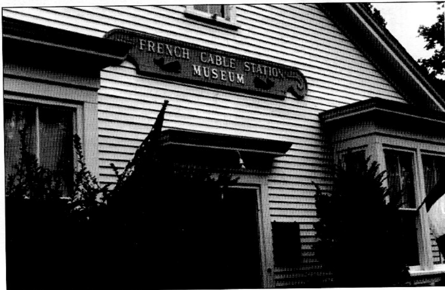
The Cable Station building is a small clapboard house on Rt. 28 in Orleans. When open in the summer, the entrance is flanked by the U.S. and French flags.
